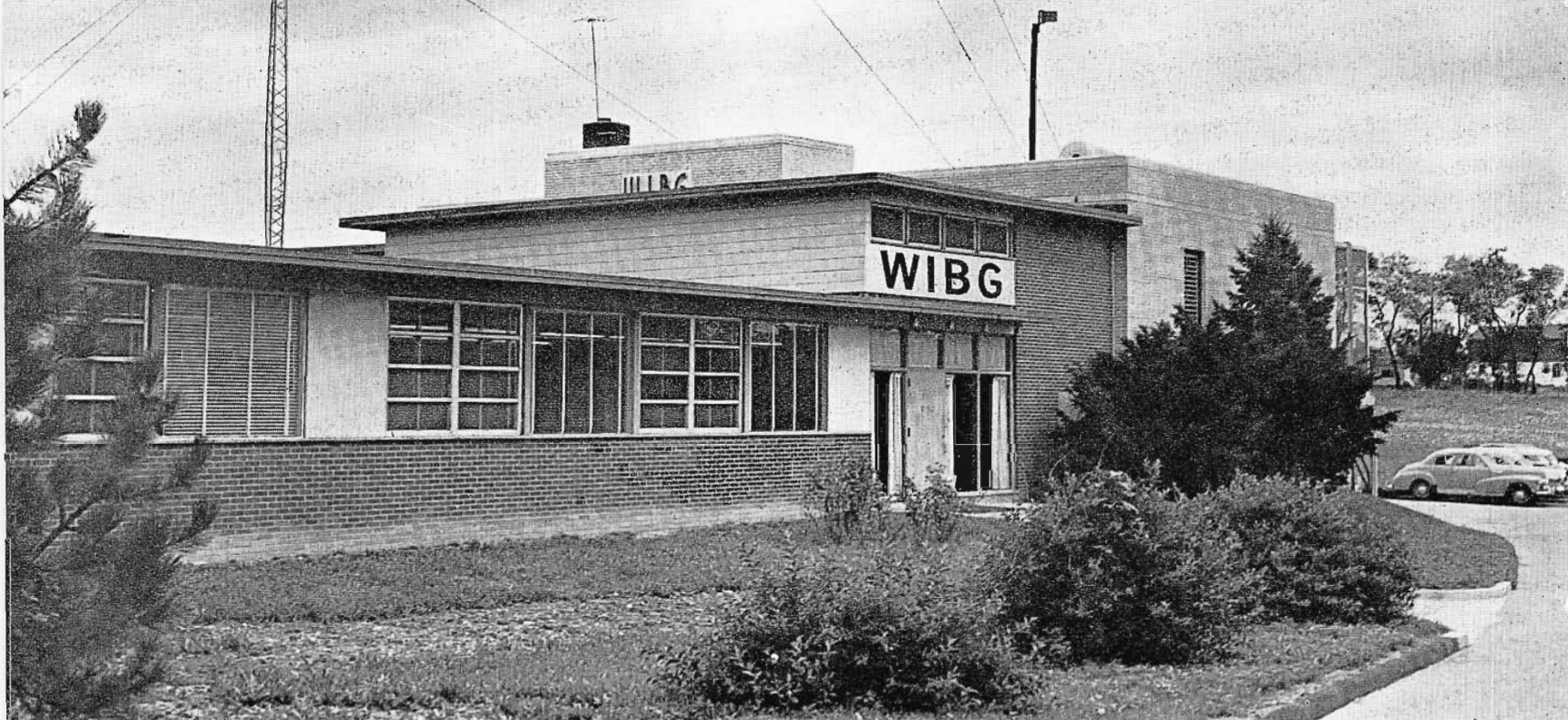
FIG. 1. WIBG's modern split level building located near Lafayette Hills in suburban Philadelphia shown here. The single story section (on the left) houses the station's offices. The larger section on the right contains the studios, control room, transmitter workshop, and garage.
