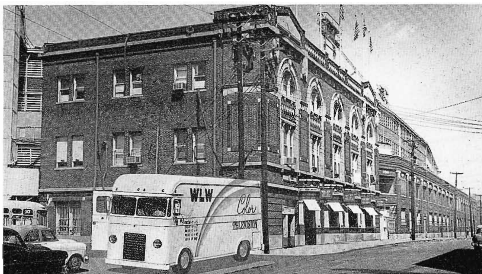
FIG. 3. The WLW Color Television Mobile Unit is parked just outside of Crosley Field. About 500 feet of camera cable connect each of the color cameras to their respective control positions located within the unit. The video switcher and audio console are also located in the unit.
